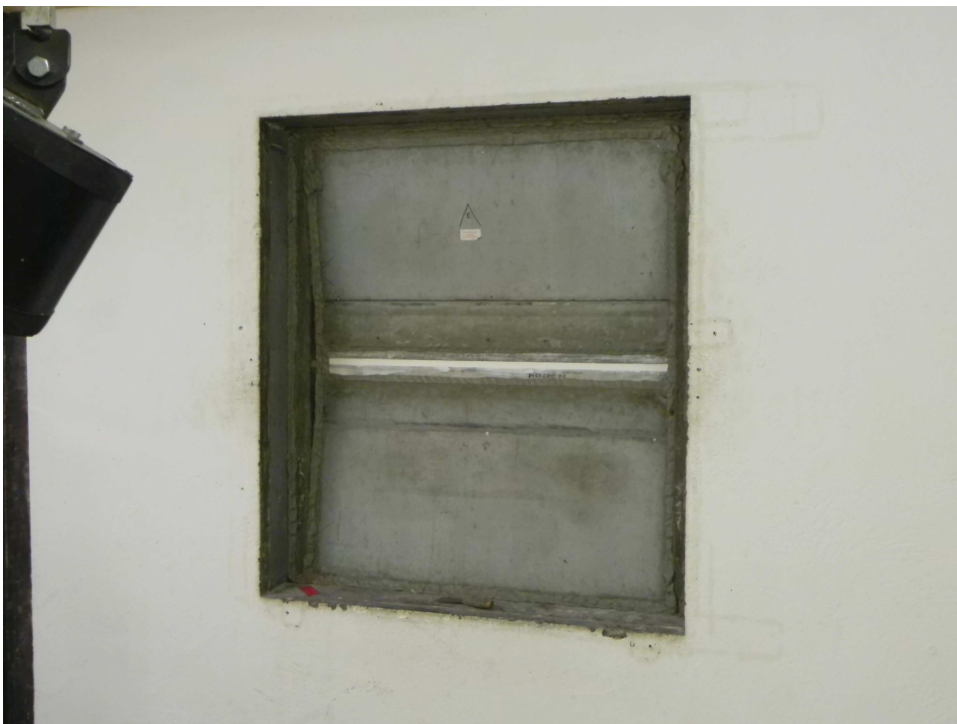
Fig. 3 Photo of the mounted element (taken by ift Laboratory for Building Acoustics)
